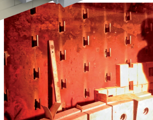
JuSys ® CFB adiabat anchor fixation and insulation
