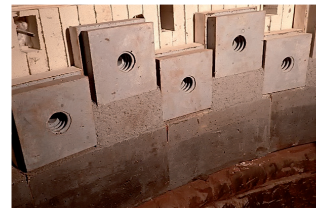
JuSys ® CFB adiabat during installation
