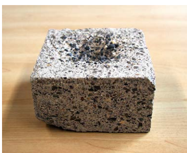
conventional LC shotcrete
