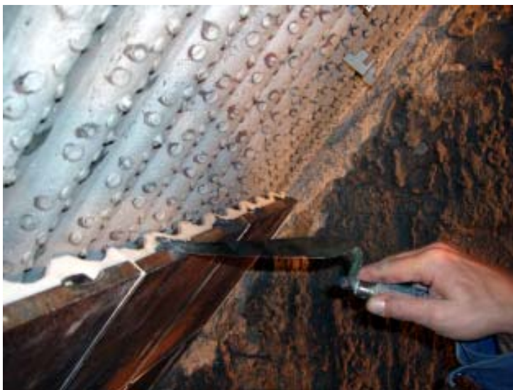
Picture top left and right Inserting the tube wall tiles
