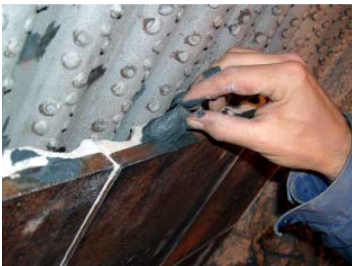
Picture left Inserting the in SiC mastic dipped SiC shaped parts as upper closing of the recess
